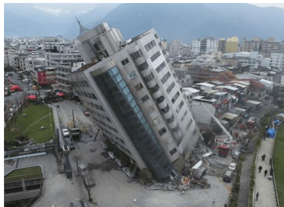
Figure 36 Soil liquefaction
