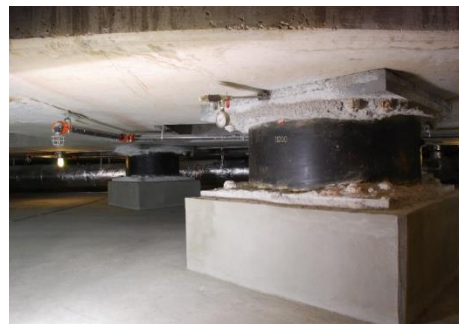
Figure 61 Base isolation
