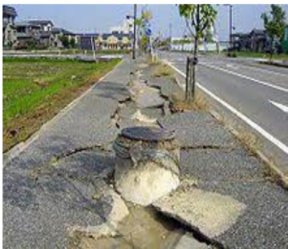
Figure 35 Soil liquefaction on road
