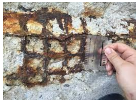
Figure 40 Chloride induced corrosion
